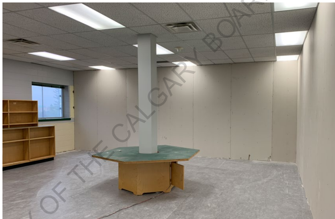
Temporary decanting space
