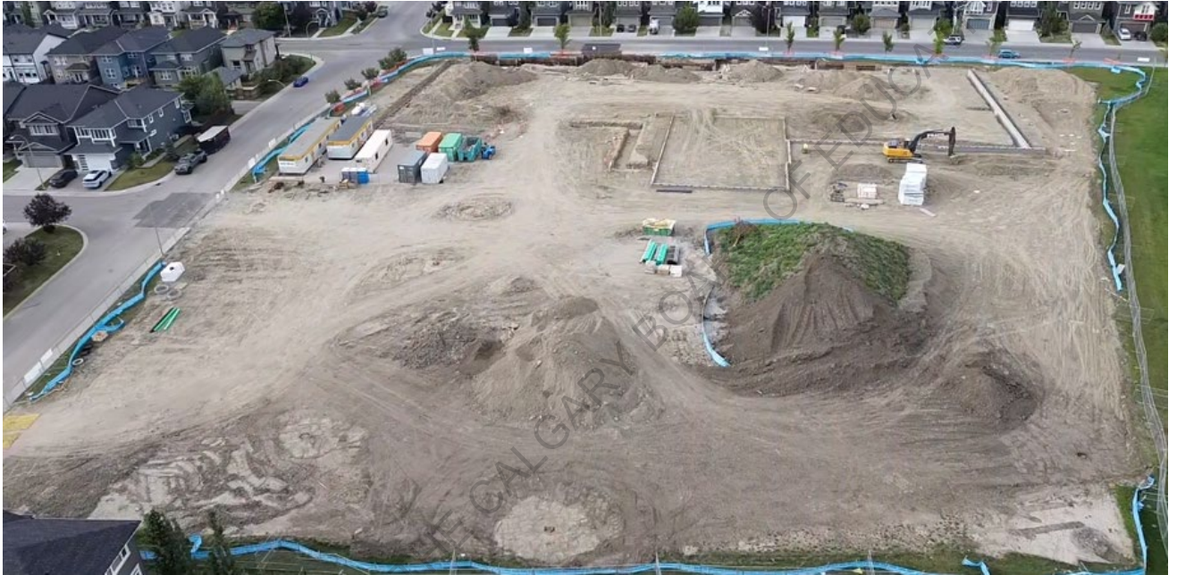
Site clearing and Foundations
