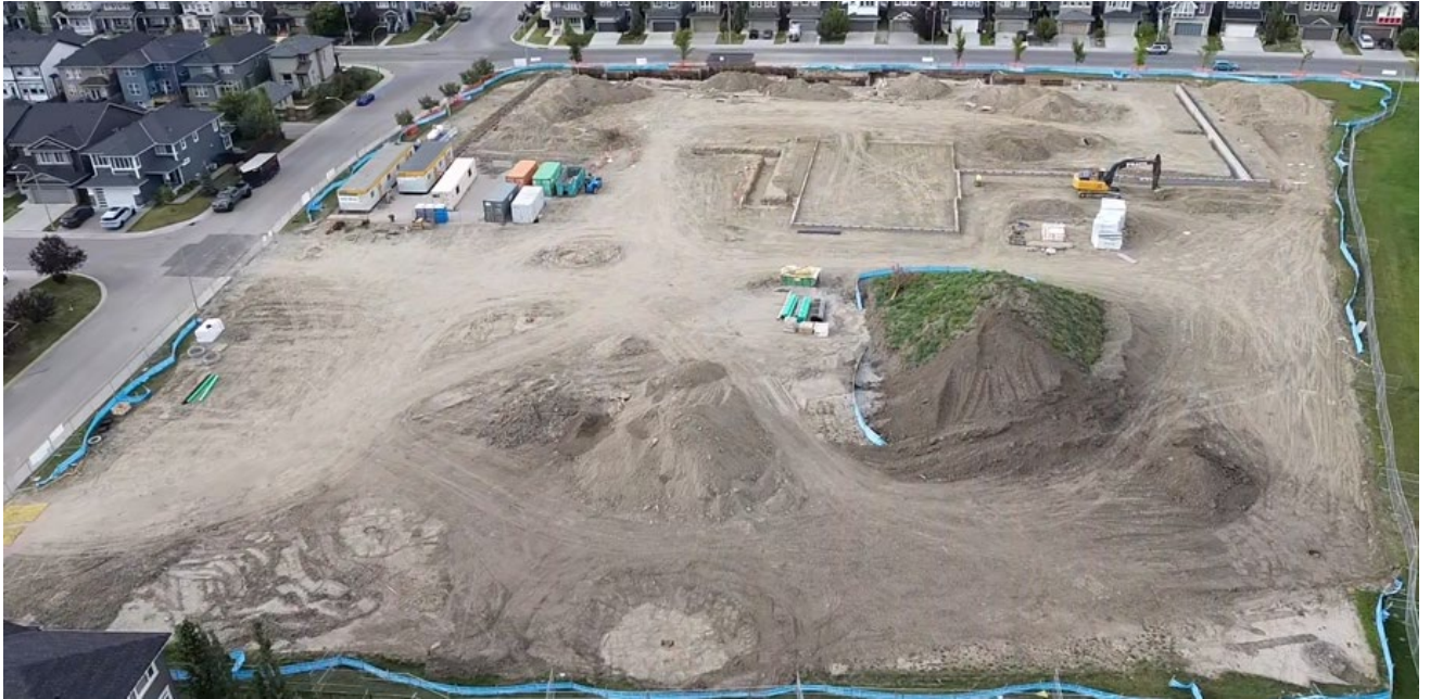
Site clearing and Foundations
